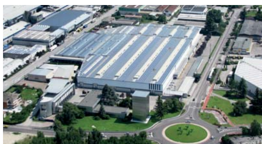
ROVERETO - TN - PREMISES AERIAL VIEW
